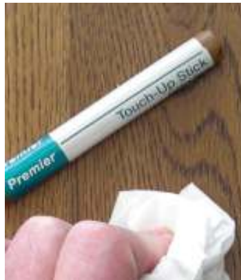
buff off excess with a soft cloth
